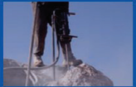
1. Drill holes into the rock & clear.
